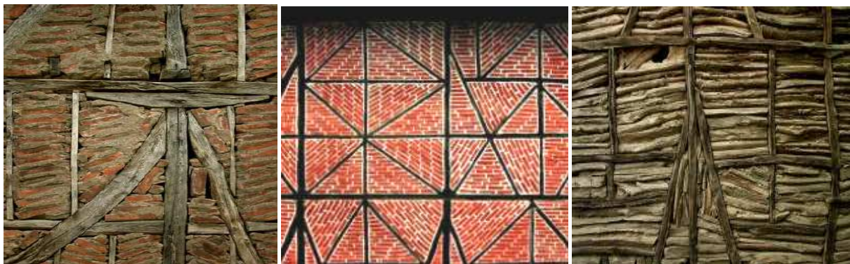
Figure 6: To the Left Hatil, Turkish Traditional Construction; in the Center Detail of the Variation Decorated with Construction Himis near Düzce; the Right Detail of the Wall Bagdadi to Golcuk [6]
